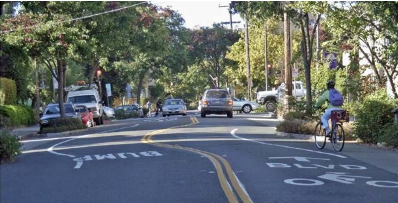
c. *Advantages.* The snake-like alignment and the lane narrowing result in lower speeds provide parking protection, shorten pedestrian crossing distance. With landscape enhancements, improves aesthetic value of street.
